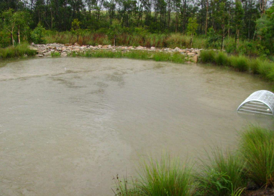
solution: sediment pond protects macrophyte zone
