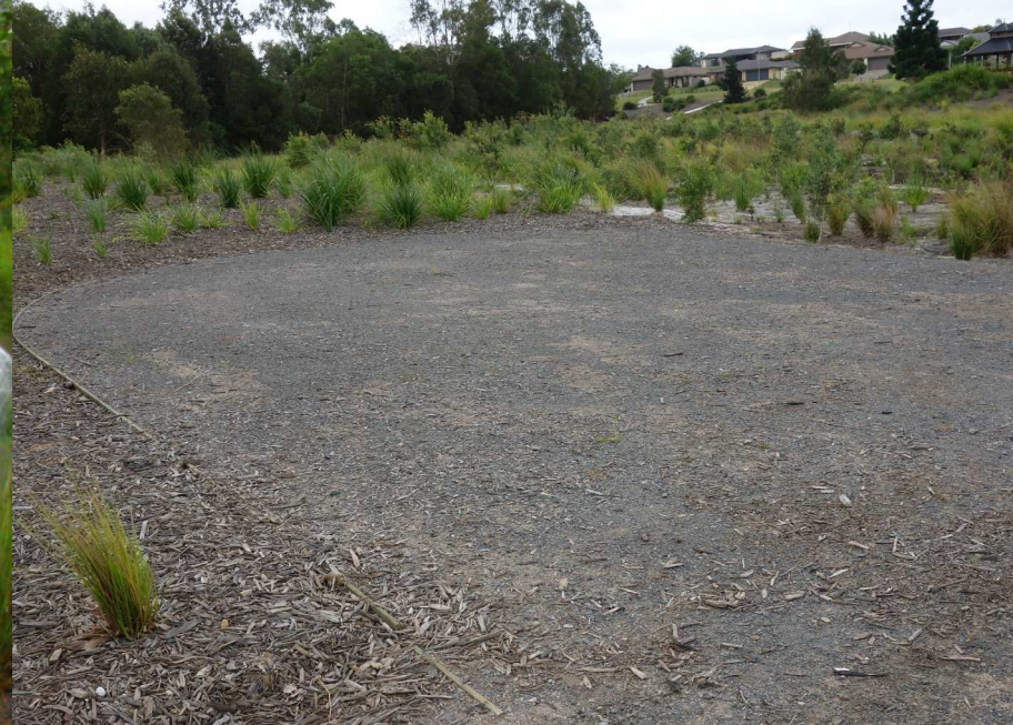
solution: silt handling and dewatering zone
