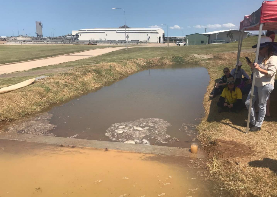
solution: high efficiency sediment basins
